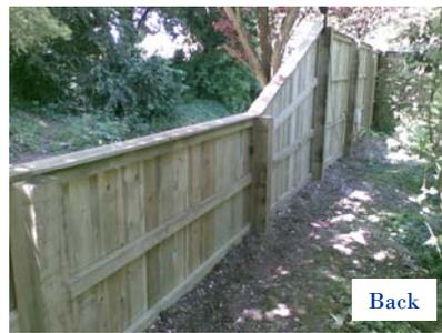
The human ear hears a halving of sound for every 10dB Sound Reduction. To put that into context normal conversation is around 60dB, heavy traffic is around 80dB. We've had our acoustic fencing checked in non-laboratory conditions and we believe there is an 8dB reduction. That's a tangible reduction on a fence installed on site doing what it's meant to do.
